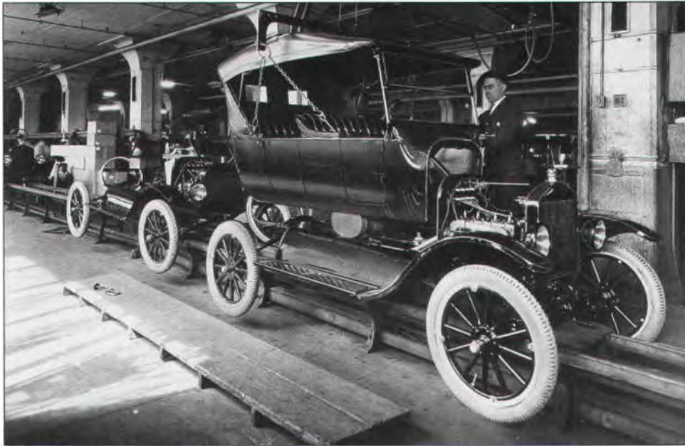
The age of the automobile had arrived. Model T Fords roll along the assembly line.
