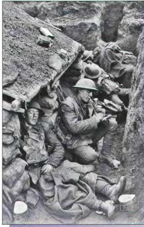
Soldiers huddled in the trenches, sometimes sleeping sitting up.
