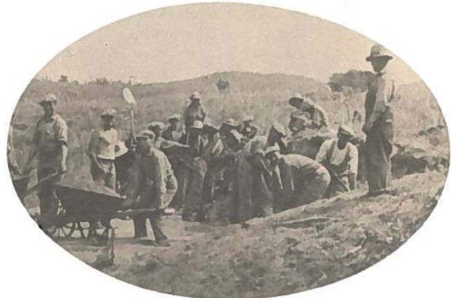
Digging a filling on a spur, Dundurn, Saskatchewan
