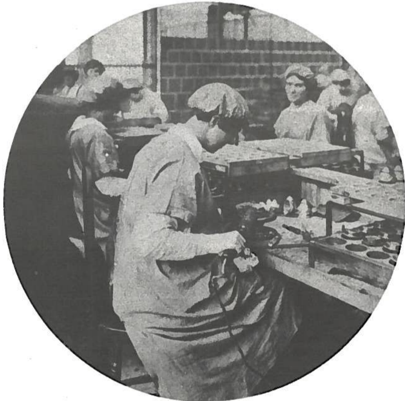
Women excelled at doing meticulous work. Here they are soldering the cap of a No. 80 fuse.
